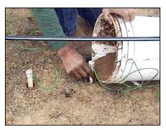
Pouring "mud slurry" made from removed soil and water.
